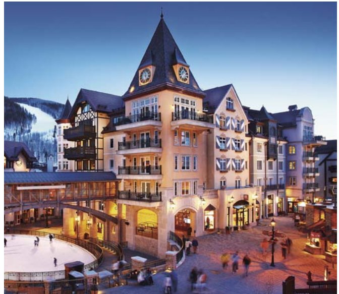
Image 33. Distinctive roof lines are created with roof forms and building heights that vary.
