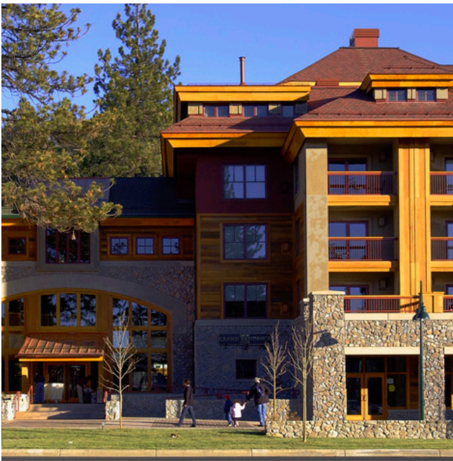
Image 30. Varying wall planes reduces the visual scale of a structure and helps to highlight interesting building features.
