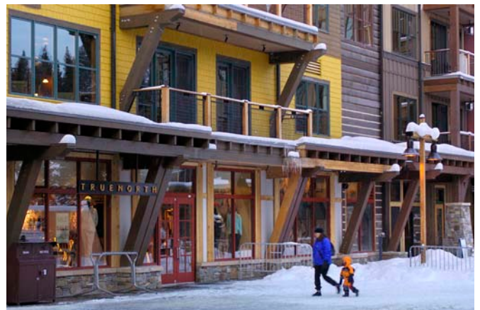
Image 19. Protruding overhead canopies create interesting architectural façades and provide protection from falling snow.
