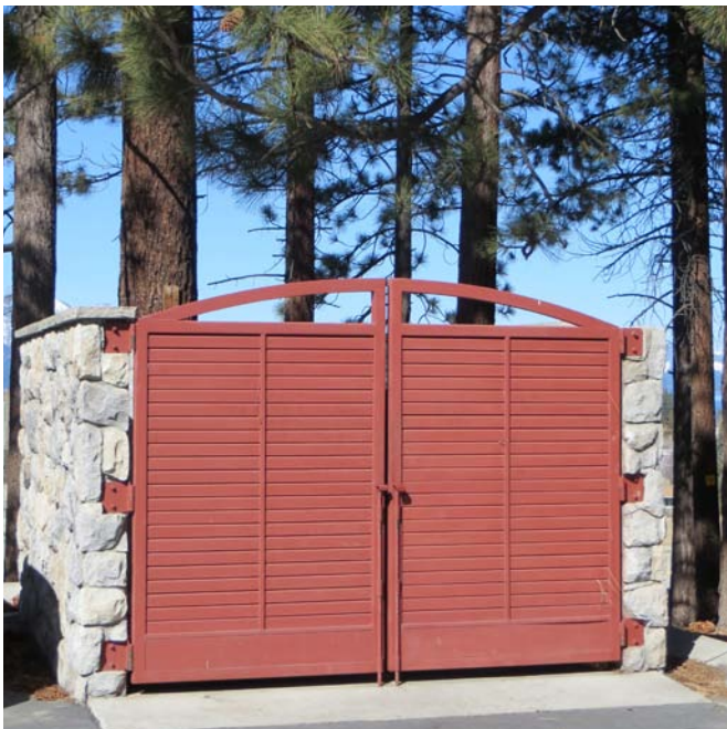
Image 43. Dumpster enclosures designed using materials and finishes consistent with the primary building helps to protect visual quality by unifying the appearance of site structures.
