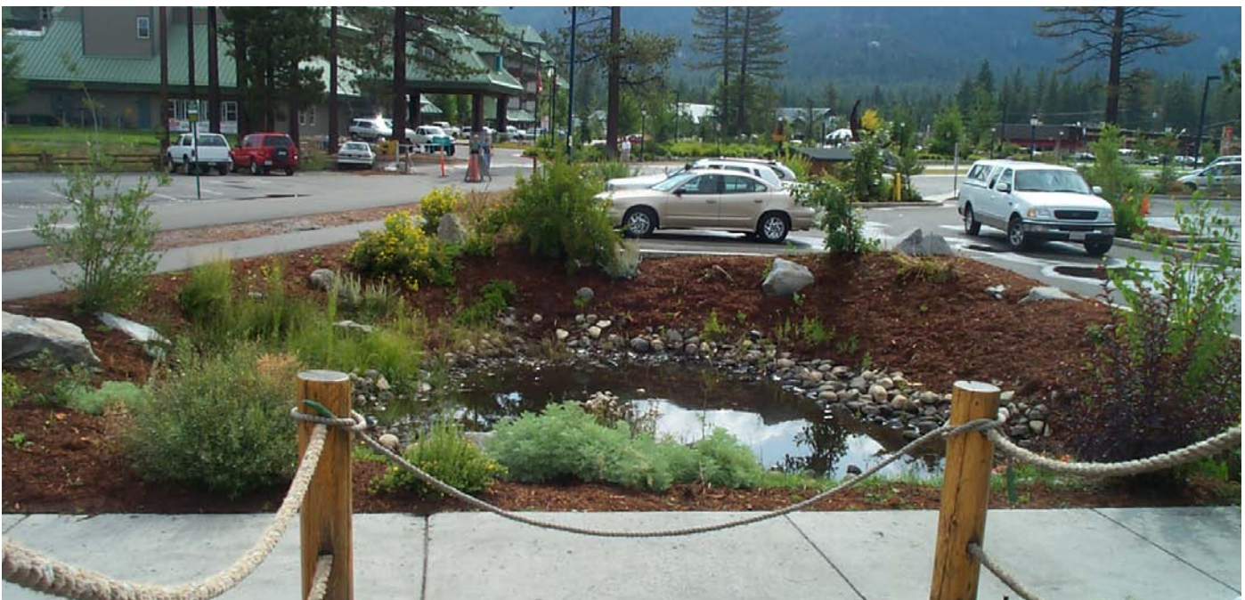
Image 13. Best Management Practices (BMPs), such as infiltration basins, provide an aesthetically pleasing and lower cost alternative to conventional storm water treatment strategies.
